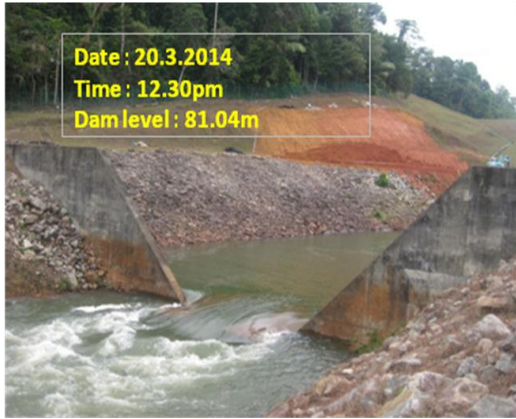
Figure 7: Flow over a Sharp Cress Weir of Juaseh Dam
